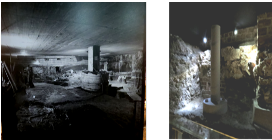
Fig. (7) The underground museum in Kraków when begin to intervene and consolidation the roofs
