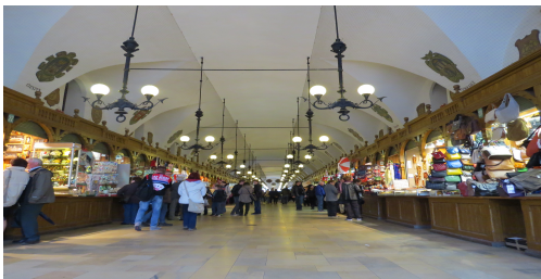
Fig(11) New light system in the shops within the Cloth Hall building, Krakow
