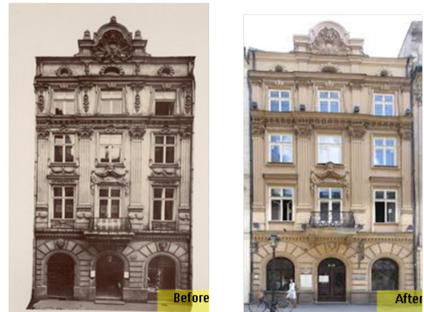
Fig. (5)The façade of Jan Matejko house before and after restoration and preserve the identity and authenticity
